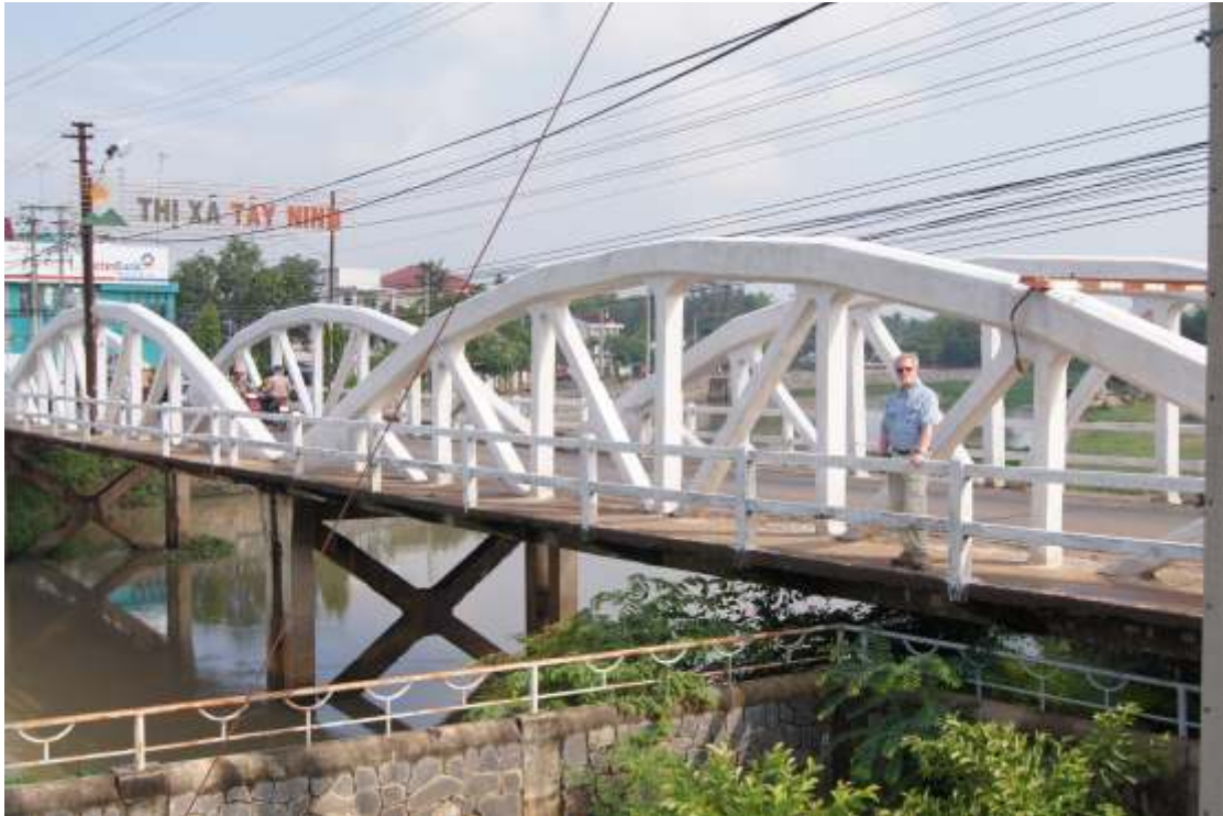
Ken stands on the Tay Ninh bridge.
